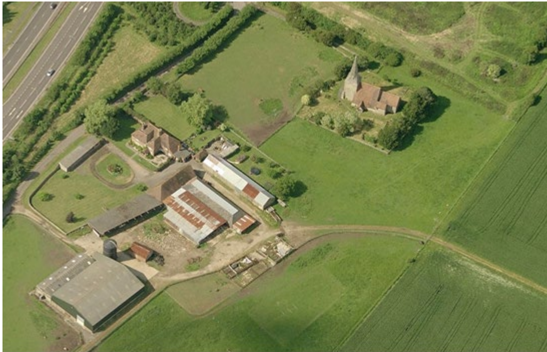
Figure 7 Court Lodge Farm farmstead with Grade 2 listed buildings and St. Mary's Church Grade I listed
